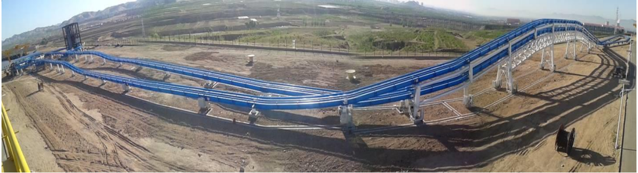
Fig. 4. A new 3rd-generation 1km-long MagTrack demoline in Zhangjiakou, China.
