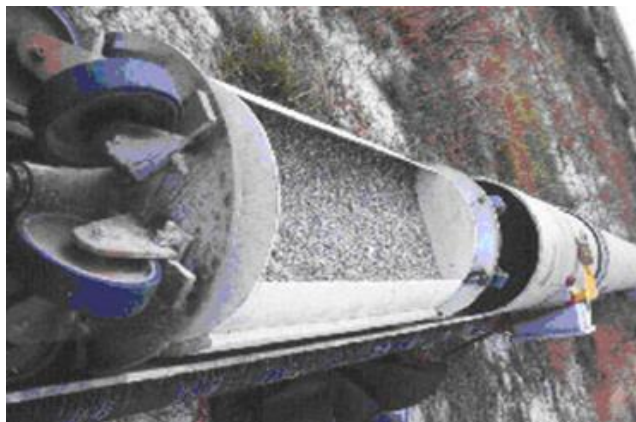
Fig. 1. A 1st-generation 270m long pipeline demoline in Lakeland, Florida.
